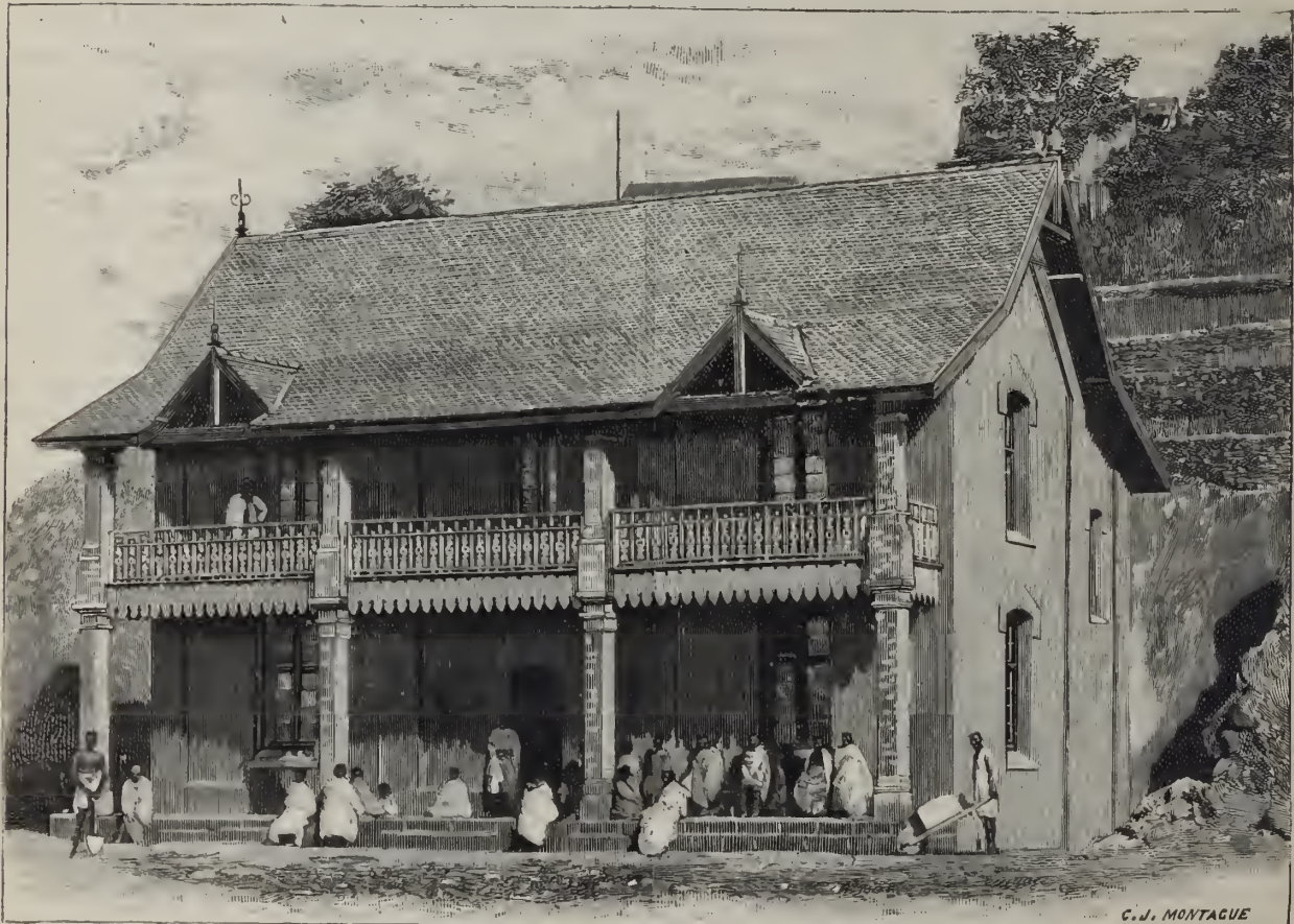
NEW COTTAGE HOSPITAL, FIANARANTSOA.
